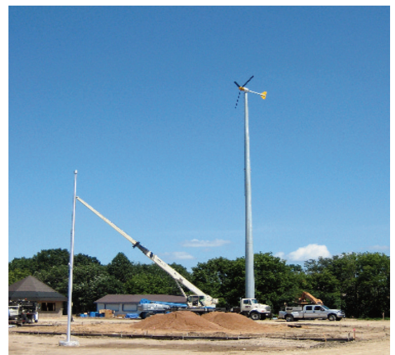
Laying the foundation for the Zephyr Wind Turbine
