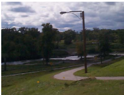
The East Grand Forks bike path is lit by solar energy.
