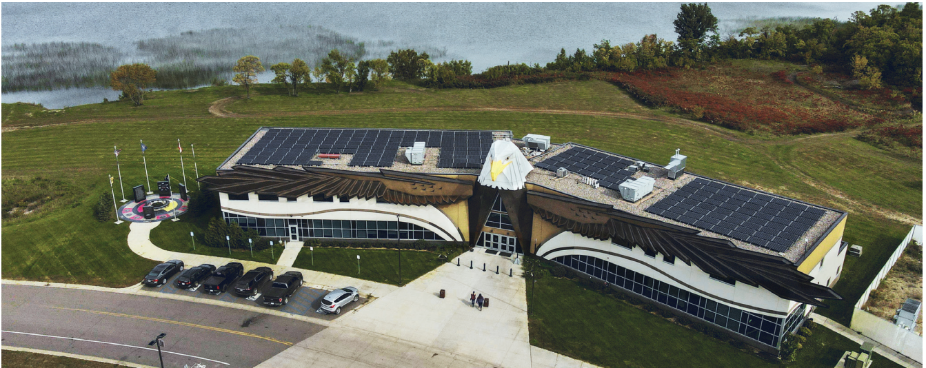
Red Lake, Minnesota. Red Lake Nation Government Center rooftop solar installation.
